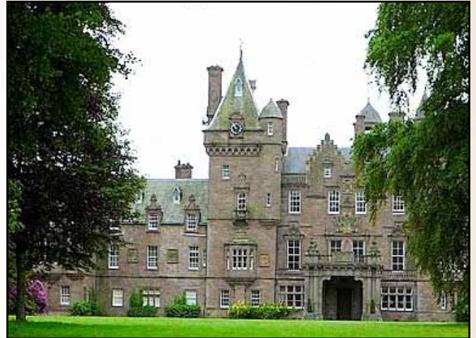
KINNAIRD CASTLE WAS DESTROYED BY TWO FIRES BUT WAS REBUILT TO ITS PRESENT CONDITION.
